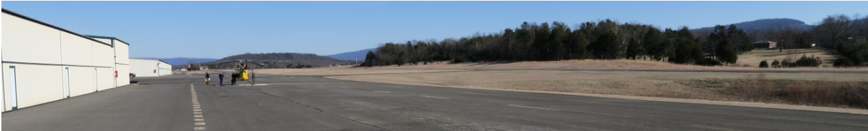
Before - looking southeast across the runway.
