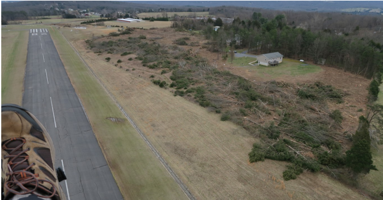
Extent of the clearing.
