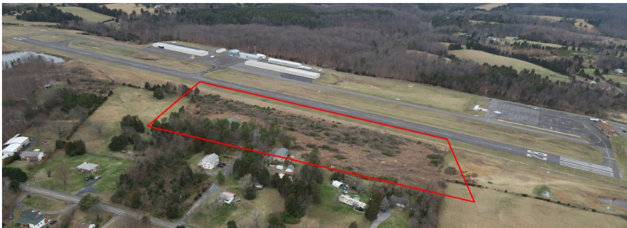
Extent of the clearing. View looking north.
