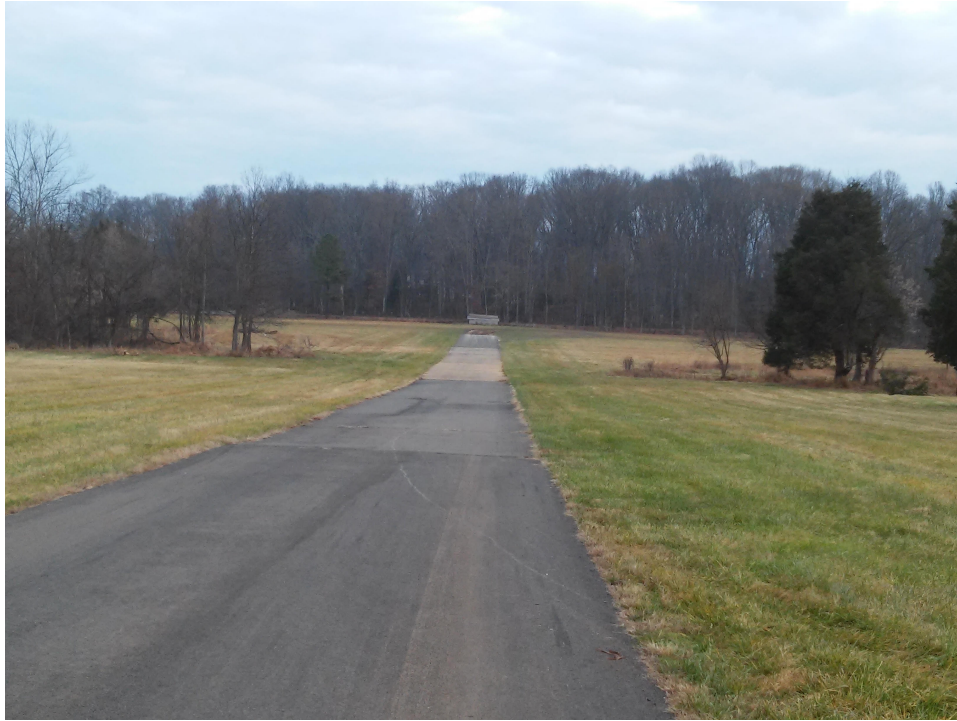
The gap before - note the trees encroaching on the left
