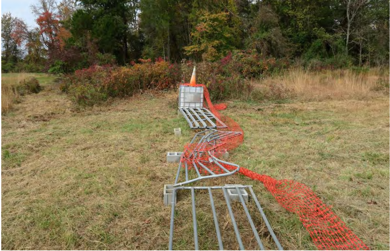
The cattle guard - improvised from fencing - showing the section that Tom hit. The section has probably been put back into place upside down since the accident since he approached from the left.
