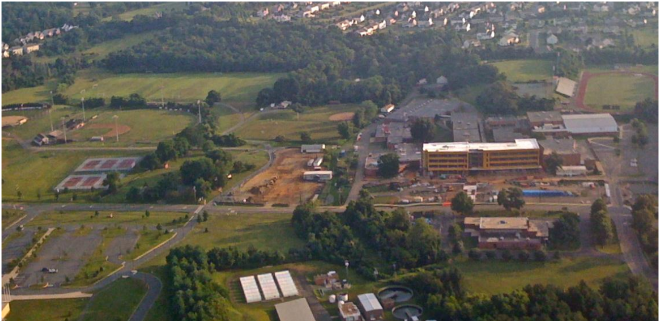
Construction on Fauquier High School in Warrenton, taken by Sierra Aceto from the back of Jay Aceto's powered parachute.
