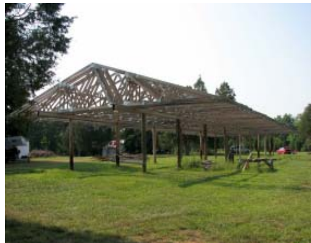
Hangar Under Construction
