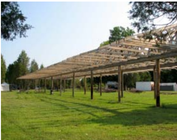
Hangar Under Construction
