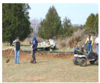
I could see across the main runway toward the two new storage buildings there and see the work crew actively engaged near them. After walking across the runway, I saw that they were engaged in digging a drainage ditch and laying flexible hose in it. I remember Tom telling us how he planned to draw some of the moisture away from the southern end of the field.
